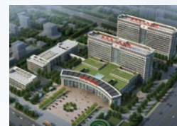
Guan County People's Hospital Relocation and Complex Construction Project
