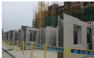
Anyue Jiayuan Residence Affordable Housing Project (Phase I) Construction
