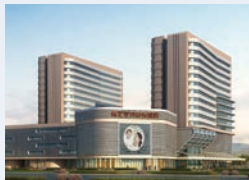
Baoding City Maternal and Child Health Hospital Relocation and Construction Project
