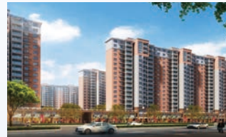
Hong Tai Court F District Affordable Housing Project
