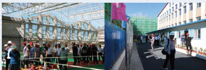
Standardized Safe and Civilized Site Observation Tour in Hohhot City
